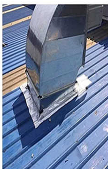
Joint Leakage
